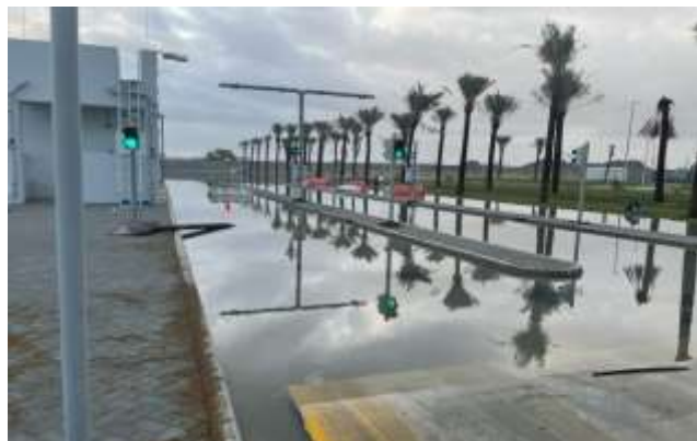
Vehicle weighbridges were completely submerged.
