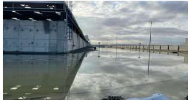
Site roads were flooded and impassable during the storm.
