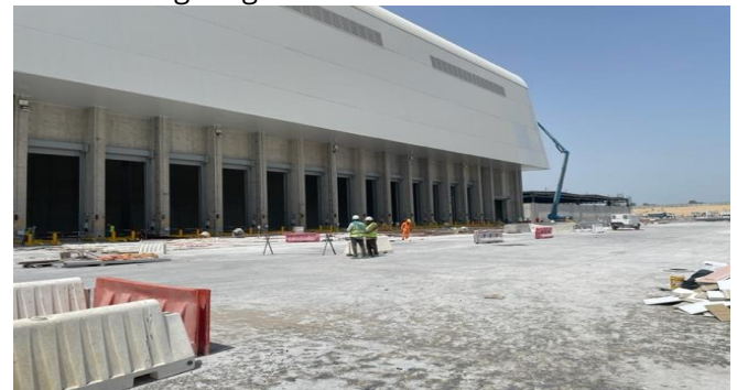
Block 2 tipping floor nearing completion
