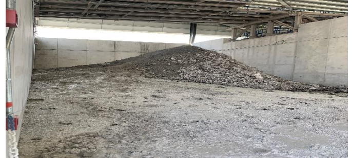
IBA recovered from the combustion process is transferred via conveyor belts into the pre-maturation area
