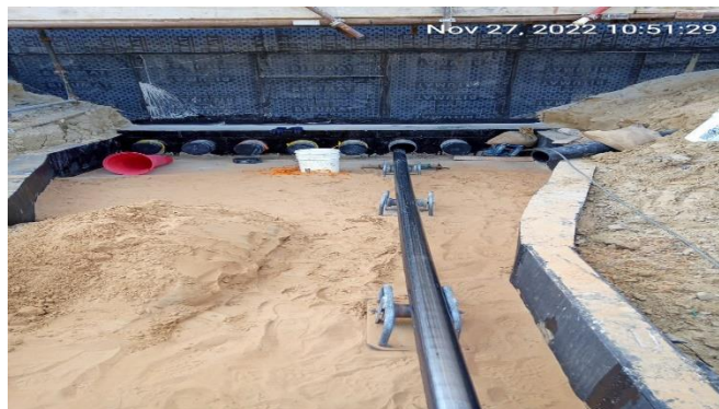
The final section of 132kv cable trench approaching the DS217 Substation
