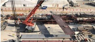
Assembly of structural steels in the air-cooled condenser has begun and primary foundations for the accommodation building have been cast. Large volumes of spoil have been removed from the eastern aspect of site near to the main entrance and grading and compacting of roadway subsurface is well underway in this area.
